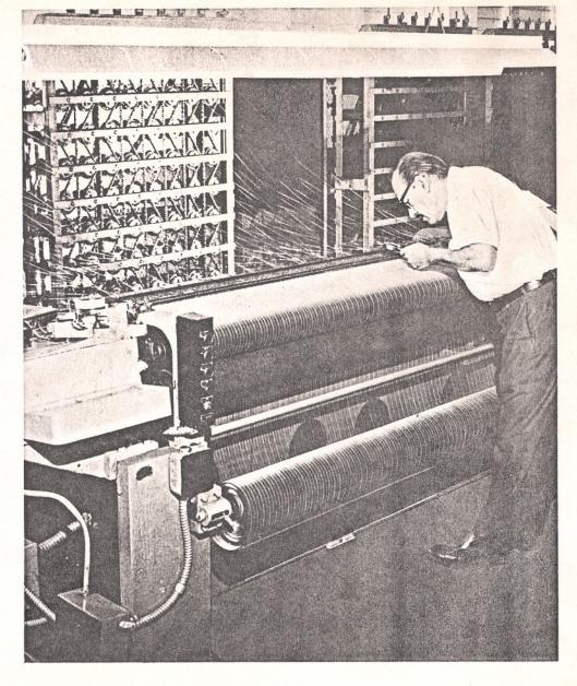
The Energy Shortage. We began preparing for this situation nearly 40 years ago when we developed an automatic weaving machine to produce the first miniature bronze louvered exterior shading device—KoolShade. Today this device is foremost on the list of effective energy-savers. A battery of these unique machines are now working overtime producing Kool-Shade Solar Screens in our plant in Fajardo, Puerto Rico—the only plant of its kind in the world.
